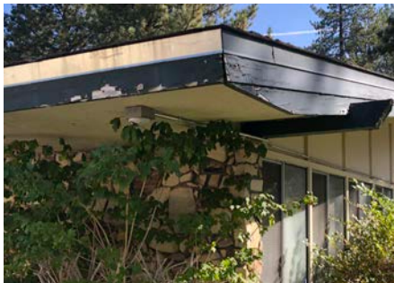
Roofing/Exterior Finish Degradation
