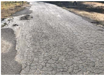
Asphalt Failing
