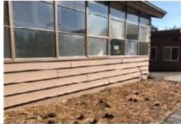
Single Pane Glazing Systems Remain
