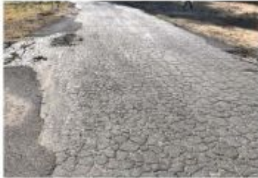
Asphalt Failing
