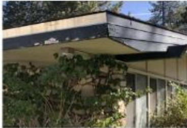
Roofing/Exterior Finish Degradation
