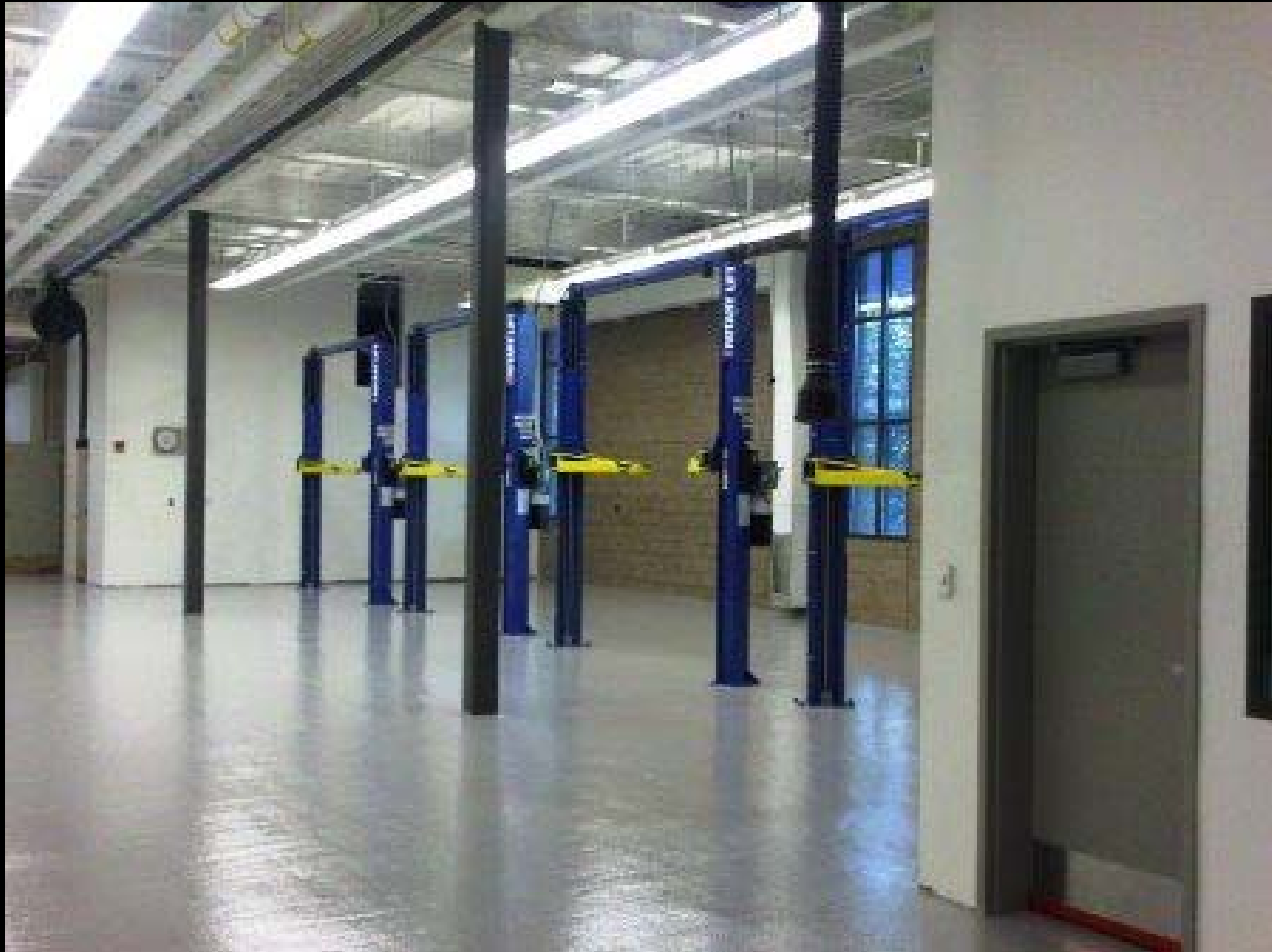
3/15/10 – CTE Auto Maintenance Bays
