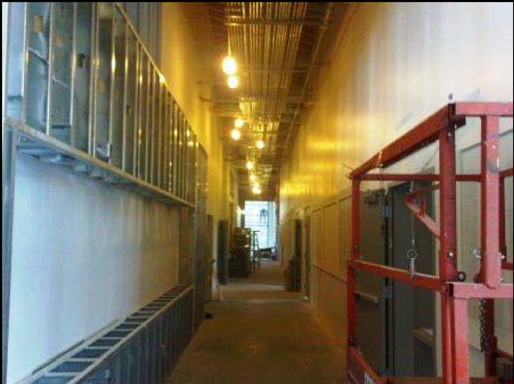
3/15/10 – CTE Classroom Corridor
