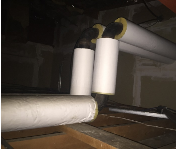
Insulation wrap with exposed insulation
