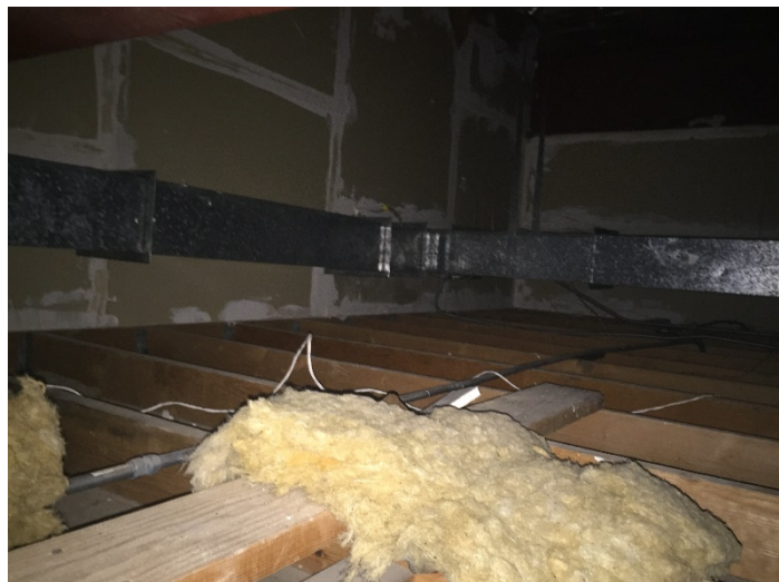
Attic space showing fiberglass insulation.
