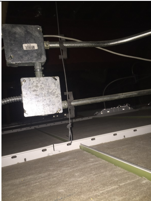
Condition in attic showing light particulates on 2x4 tiles
