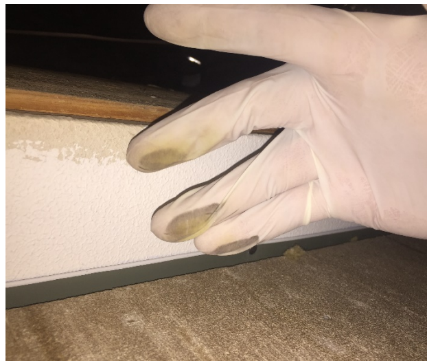
Attic space showing particulate on ceiling tiles.
